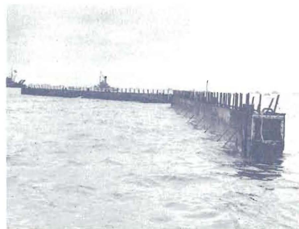
Mulberry A pontoon breakwater off Omaha Beach, 1944.
